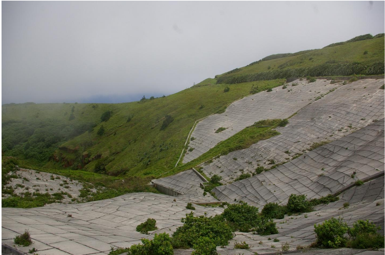
Figure 8. The head of Breakneck Valley on the southeast face of Green Mountain. The concrete was poured to facilitate capture of moisture from the southeast trade winds.
